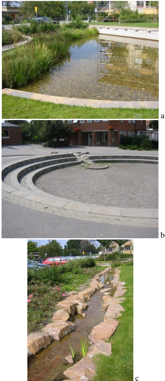
Figure 2. Stormwater system in Augustenborg: a) wet pond located between block of flats, b) dry retention basin, c) open natural channel (Photos: M. Mrowiec)
